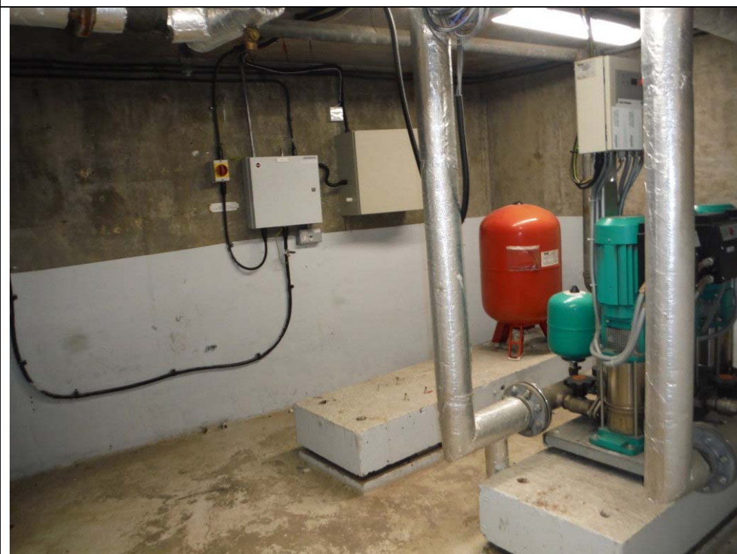
3) Apparent in-situ concrete to plant room
