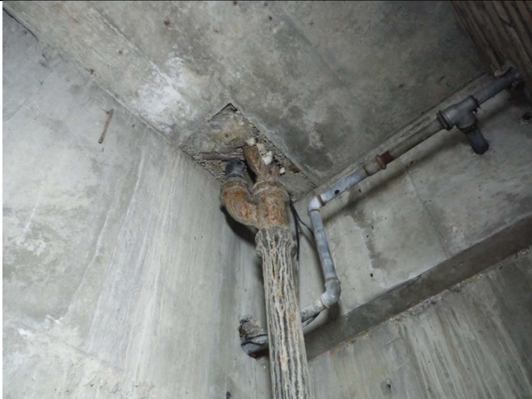
4) Apparent in-situ concrete to tank room floor and walls
