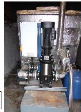
Pump set and Break Tank
