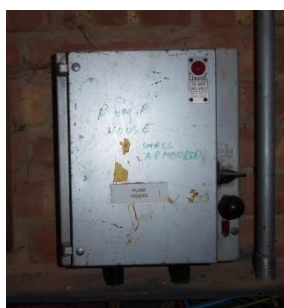
Oldest isolator serving the Booster Pump room
